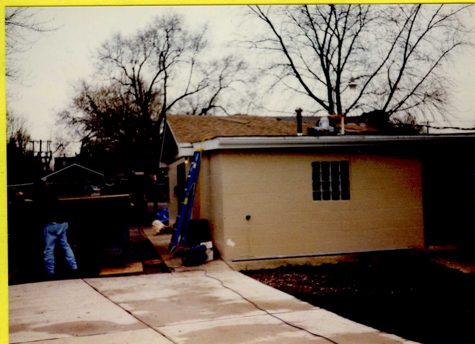
NEW SHINGLES/ROOF REPAIR - 1998
