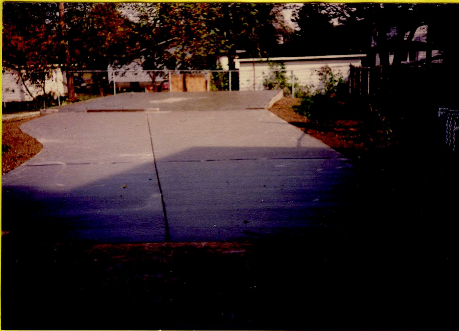
STORAGE BUILDING AND DRIVEWAY CONSTRUCTION 1995
