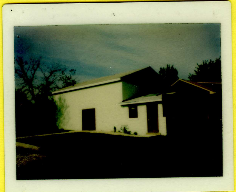
LPHOA COMMUNITY BUILDING AND WEST PUMPHOUSE VARIOUS STAGES OF REMODELING
