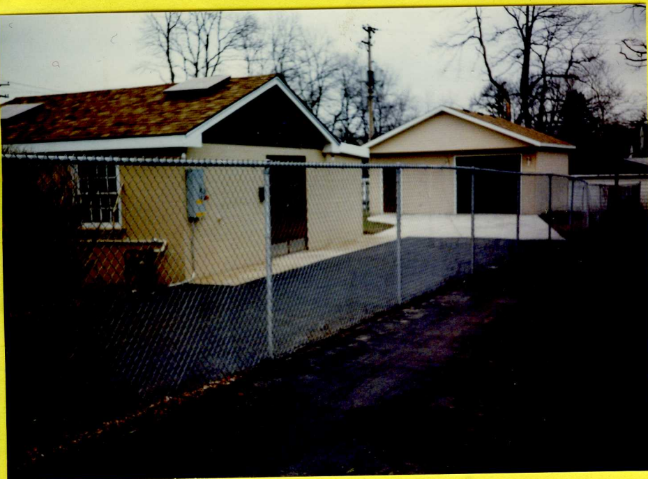
LPHOA EAST PUMPHOUSE, LAB AND CHLORINE ROOM ADDITION AND STORAGE BUILDING - 1995
